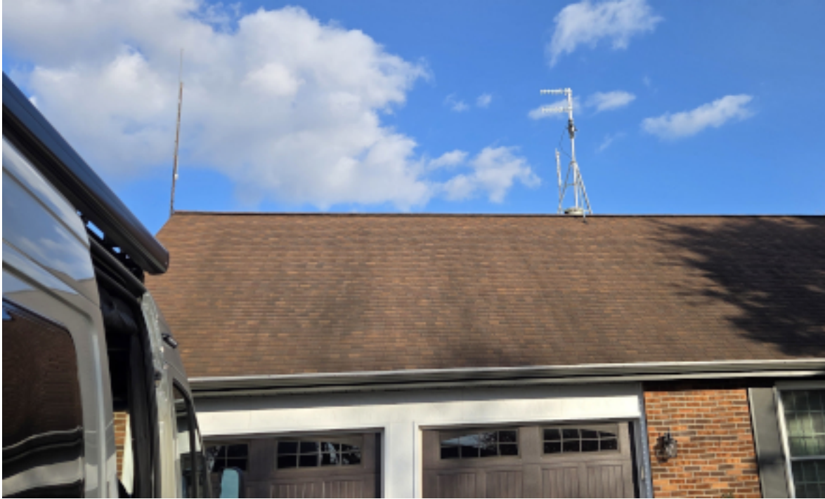
Figure 5: Good antenna placement on a ridge or rooftop
